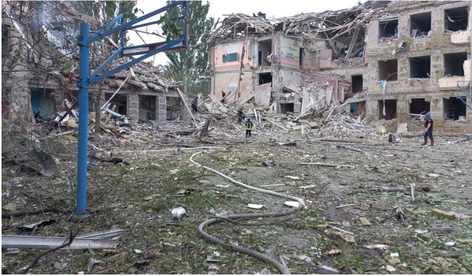
School in Kramatorsk following Russian bombardment on July 21, 2022 (Wikimedia Commons: from the website of the State Emergency Service of Ukraine – dsns.gov.ua) https://commons.wikimedia.org/wiki/File:Russian_bombing_of_a_school_in_Kramatorsk,_July_21,_2022.jpg
